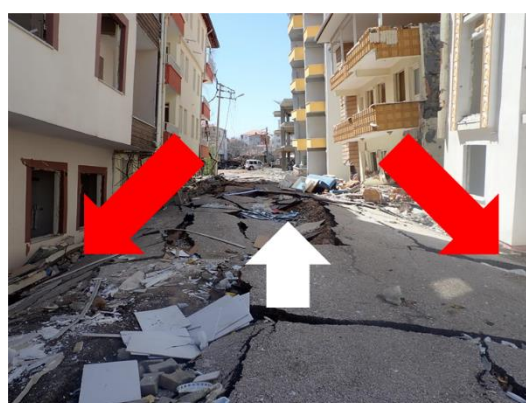
Figure 18. Road uplift and settlement / tilting damage to buildings on either side of the road
