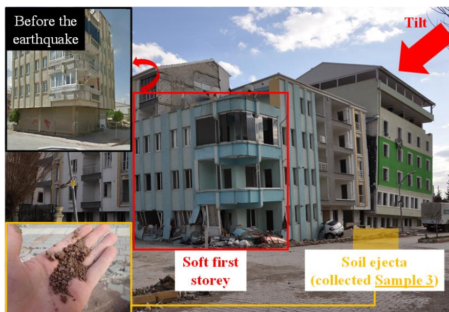
19. Structural damage (soft first storey) – blue building, and settlement / tilting damage of a building (green and white) that reportedly had pile foundations
