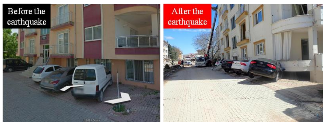
Figure 17. Building suffered from subsidence of about 1.5 m – before and after the earthquake
