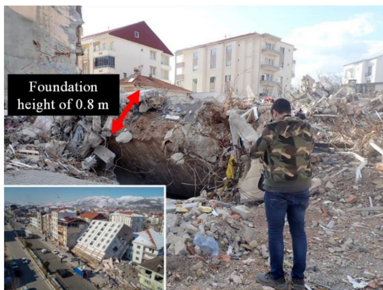
Figure 15. Tilted foundation of demolished building [5]
