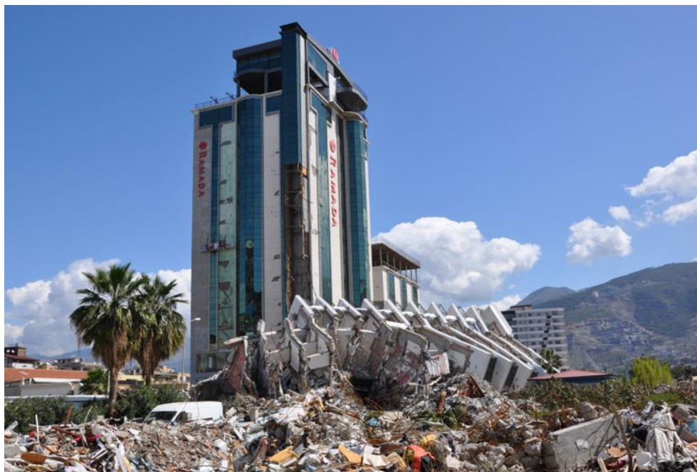
Figure 4. Collapsed building located in the former marshland – near Hotel Ramada
