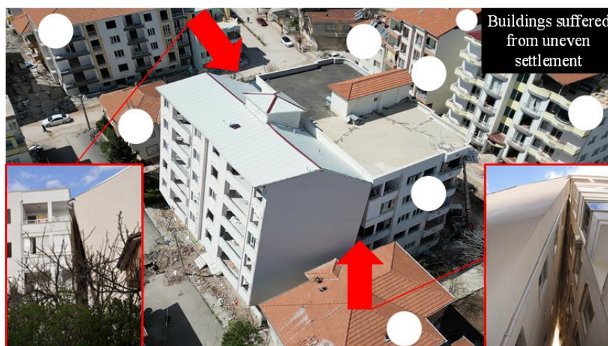
Figure 16. Heavily tilted building and surrounding buildings with similar damage
