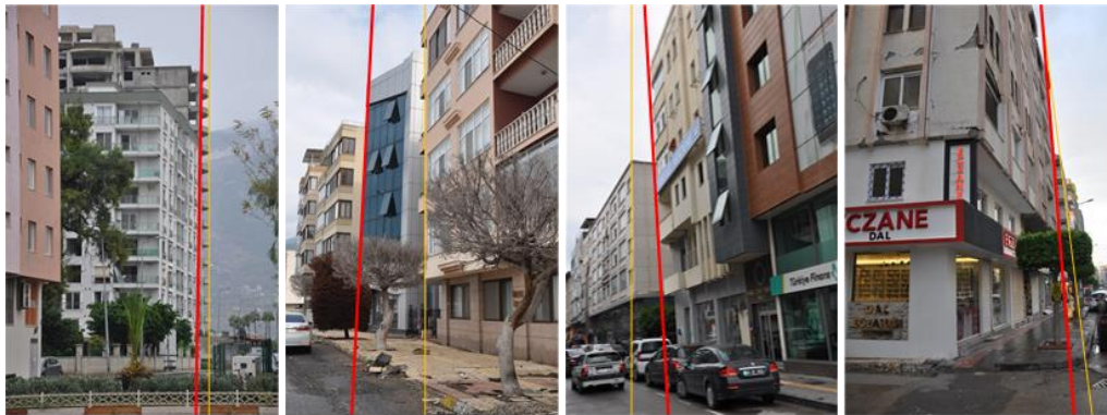
Figure 5. Tilted middle-rise buildings near the sea-coast (at the beginning of the reclaimed land)
