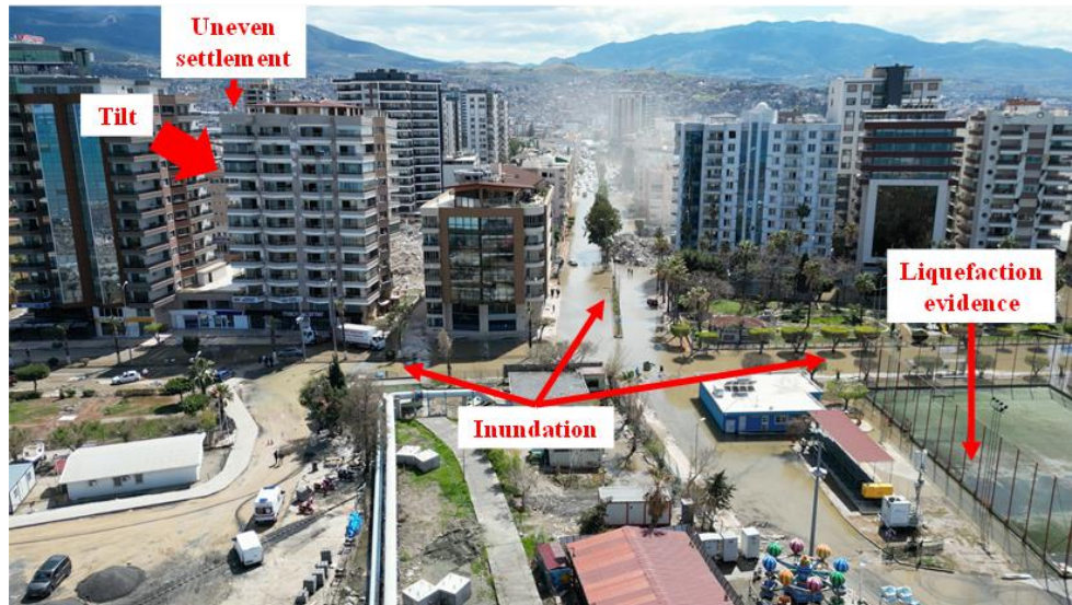
Figure 3. Evidence of various kinds of geotechnical problems observed in Iskenderun
