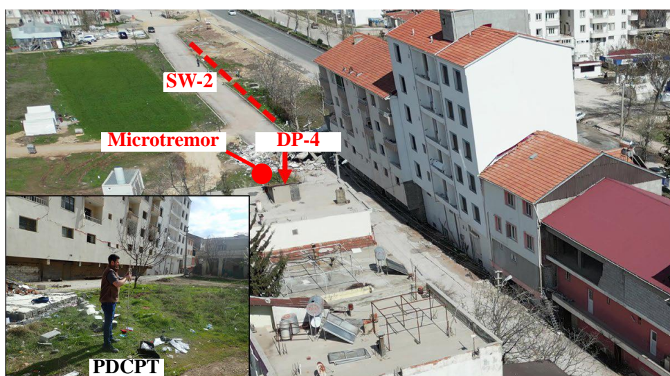
Figure 21. Locations of PDCPT, MASW and microtremor measurement conducted near buildings with subsidence / tilting damage ( 37^{\circ}47'26.57''N , 37^{\circ}39'7.88''E )
