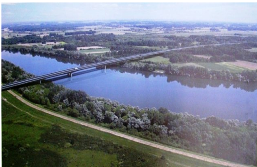
Slika 4 Most preko rijeke Save na Koridoru Vc Figure 4 River cross rivev Sava on Corridor Vc
