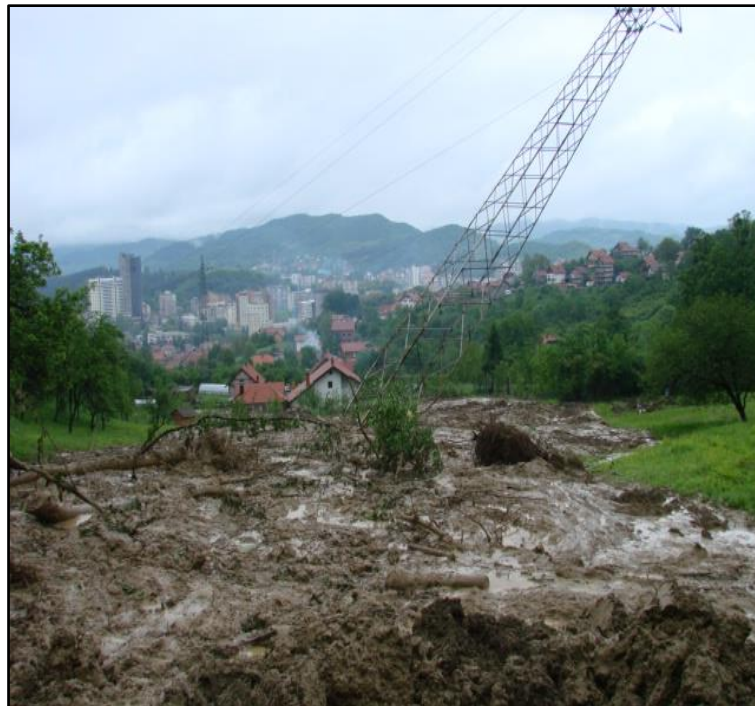
Figure 1 Ground situation after the landslide
