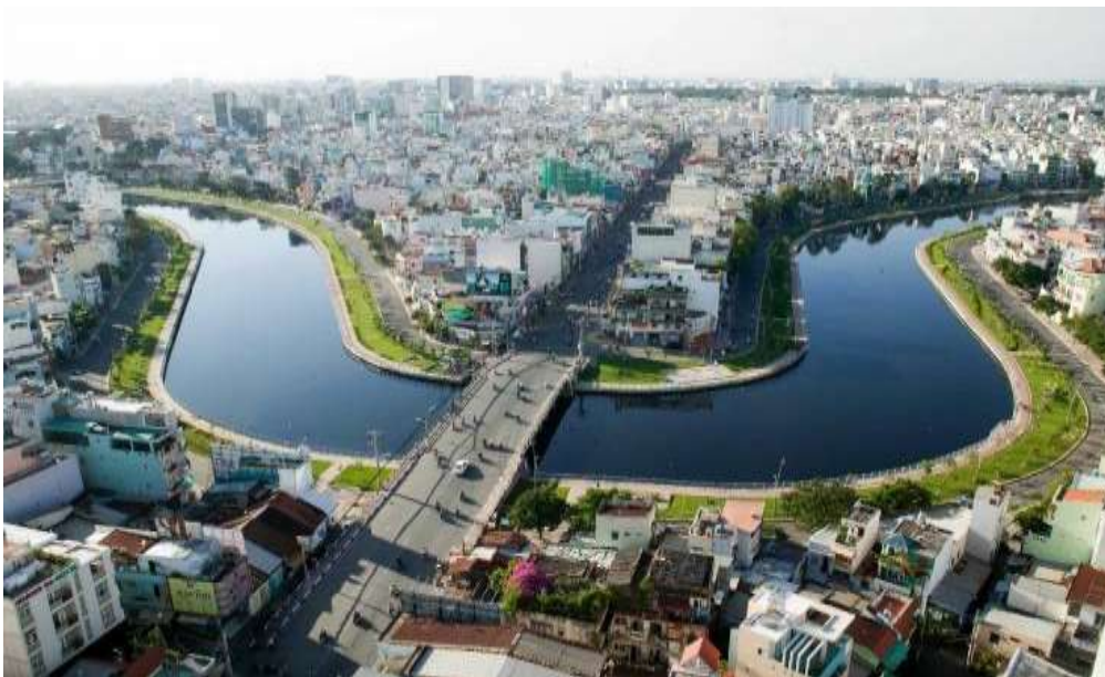
Figure 13. Nhieu Loc–Thi Nghe Canal after environmental rehabilitation and public-space improvement
